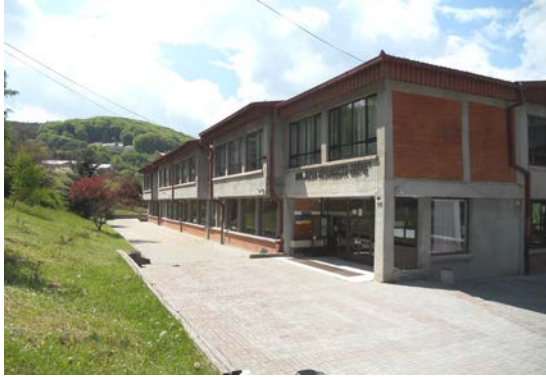
Before the renovation activities:
